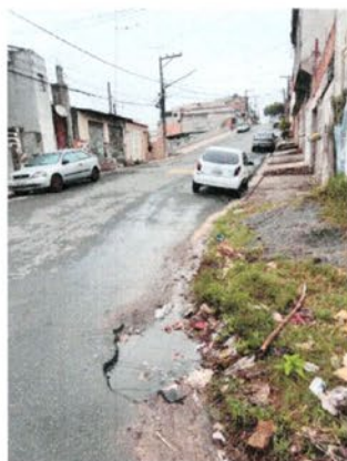
Rua José Moraes Bueno recompor o pavimento, base, guias e as setas
