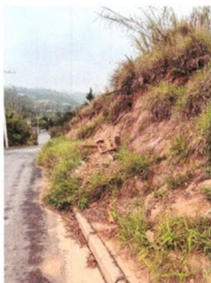
Rua João Rodrigues Dias recompor as guias, sarjetas, calçada e a talude
