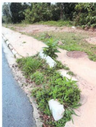
Estrada Ibrahim Tannous Abi Chedid recompor as guias, sarjetas, boca de lobo e a calçada
